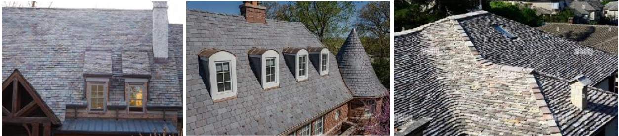
Gambar 4. Atap batu tulis (Stone slate roofing) . Sumber: Kaur, 2021
